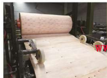
拼接后卷板机 Veneer rolling system after splicing
